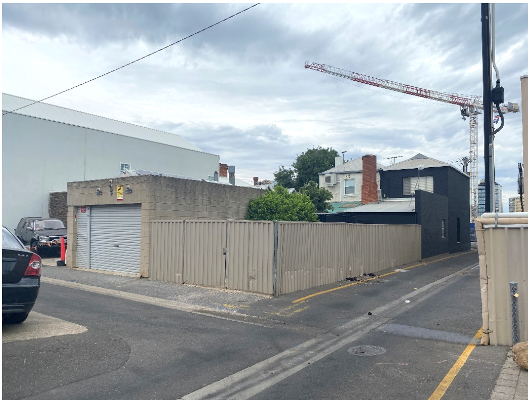
Figure 3.4 – rear of dwellings to the southeast of subject site
