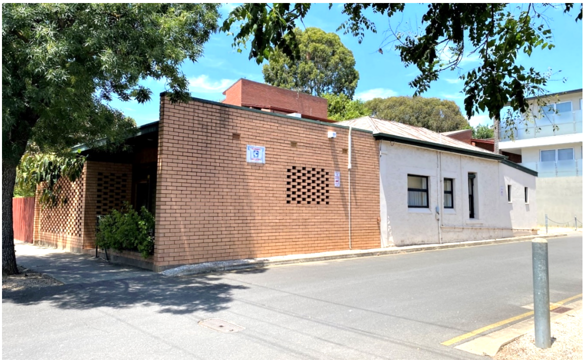
Photo 3.2 – existing building with adjacent right of way visible to the right
